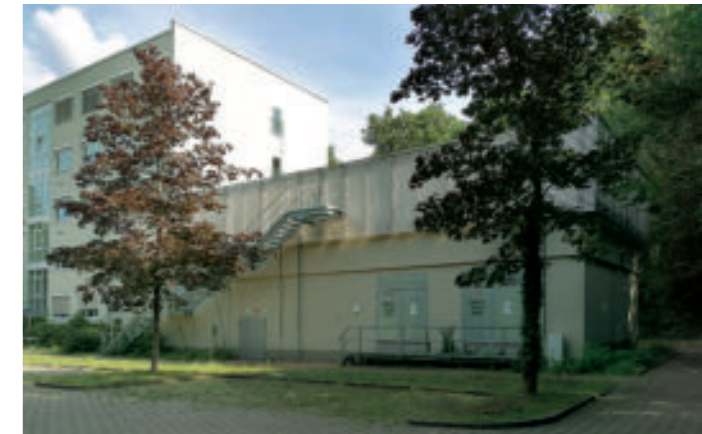
Exterior view of the former transformer building.
