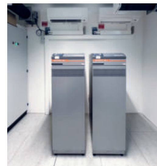
UPS systems provide a constant, uninterruptible power supply.
